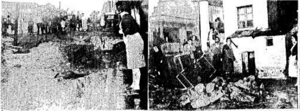
Figure 6: Disasters caused by overflowing stream in the west area of Thessaloniki. Source: Makedonia Journal, 6/12/59, p. 7
